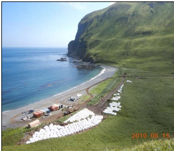
PHOTO 10 VIEW FROM HELICOPTER OF BEACH STAGING AND CAMP AREA AFTER ESTABLISHMENT OF ROAD, WITH SUPERSACKS STAGED TO BE PICKED UP BY BARGE. (2019)
