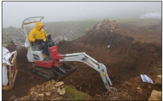
PHOTO 5 EXCAVATING CONTAMINATED SOIL WITH MINI-EXCAVATOR AT THE UPPER CAMP. (2020)
