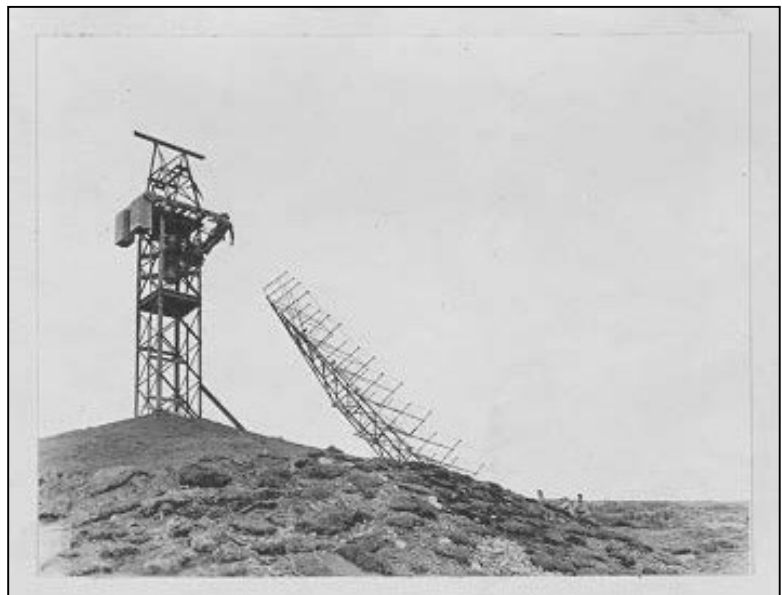
PHOTO 7 HOISTING OF ANTENNA ON DETECTOR BUILDING, 15 JUNE 1942
