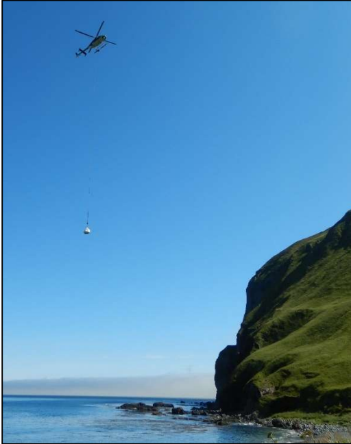
PHOTO 4. VIEW OF HELICOPTER SLINGING CONTAMINATED SOIL FROM UPPER CAMP TO BEACH STAGING AREA. (2020)
