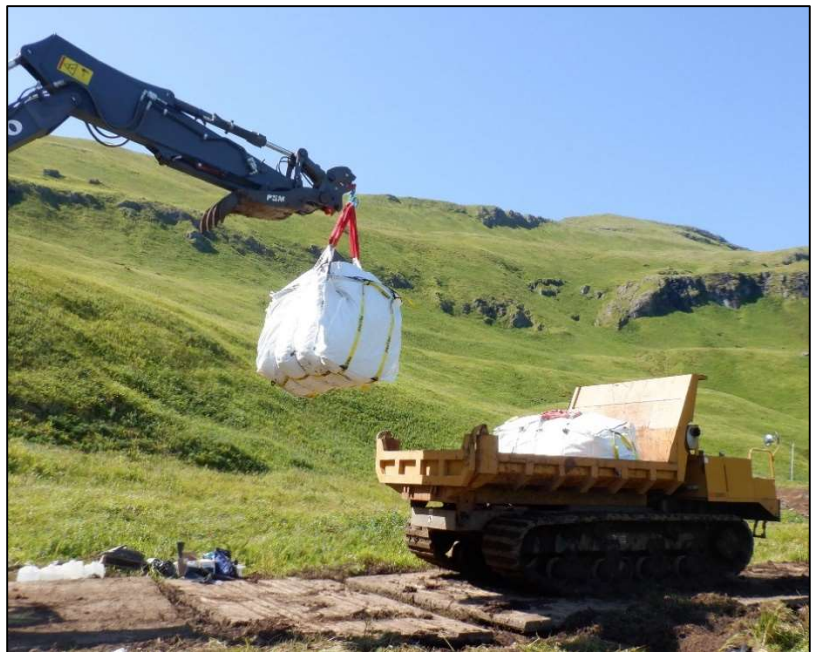
PHOTO 8 VIEW OF EXCAVATOR LOADING LOW GROUND PRESSURE TRACKED EQUIPMENT (MOROOKA®) WITH BULK BAG CONTAINING CONTAMINATED SOIL FOR TRANSPORT TO THE BEACH STAGING AREA. (2020)
