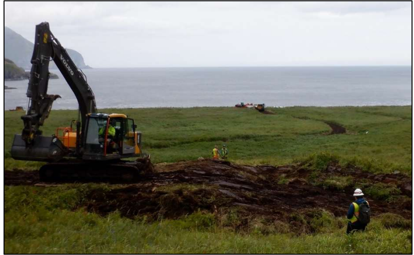
PHOTO 9 FINAL GRADING OF THE LOWER CAMP STANDBY POWERHOUSE FOLLOWING EXCAVATION OF CONTAMINATED SOIL. VIEW OF TEMPORARY TRAIL TO BEACH IN BACKGROUND. (2020)
